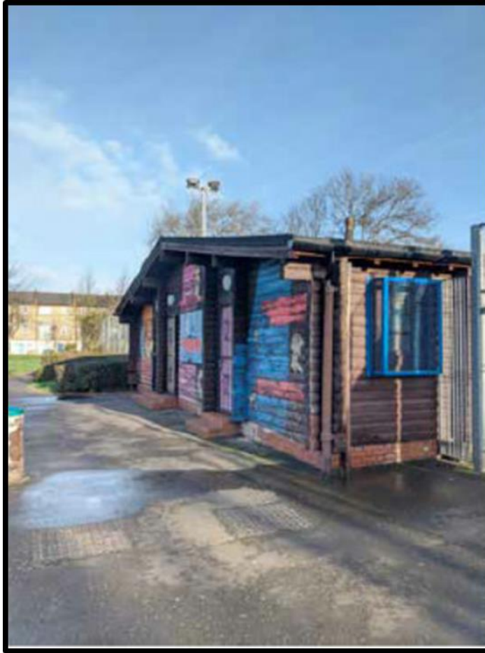
Image 5: Rear elevation of existing building.
