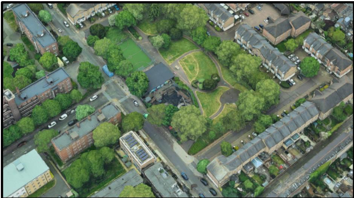
Image 2: View of site looking south.
