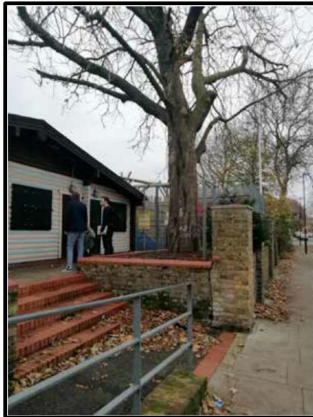
Image 4: Existing ramp and tree.
